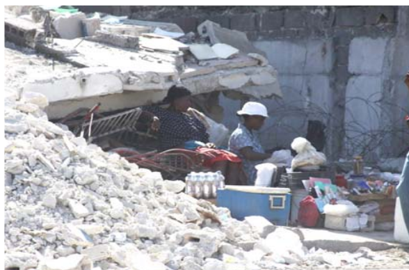
More than 250,000 residential and 30,000 commercial buildings collapsed so one million people remain homeless in Haiti.
